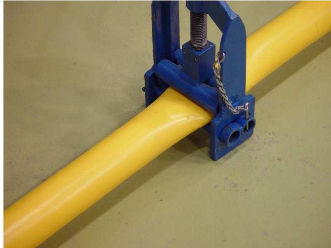
Figure 16: Squeeze-off procedure on PA12
