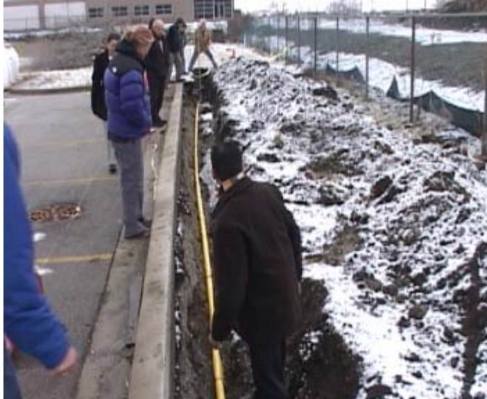
Figure 11: Installation of 2" PA12 pipe at GTI test facilities
