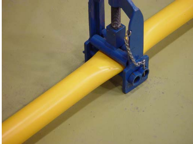
Figure 9: Application of squeeze-off procedure on PA12 pipe
