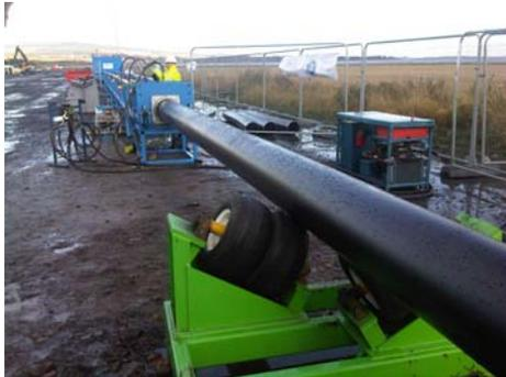
**Image Caption:** Installation of a polymer liner by the Swagelining™-Technology.
